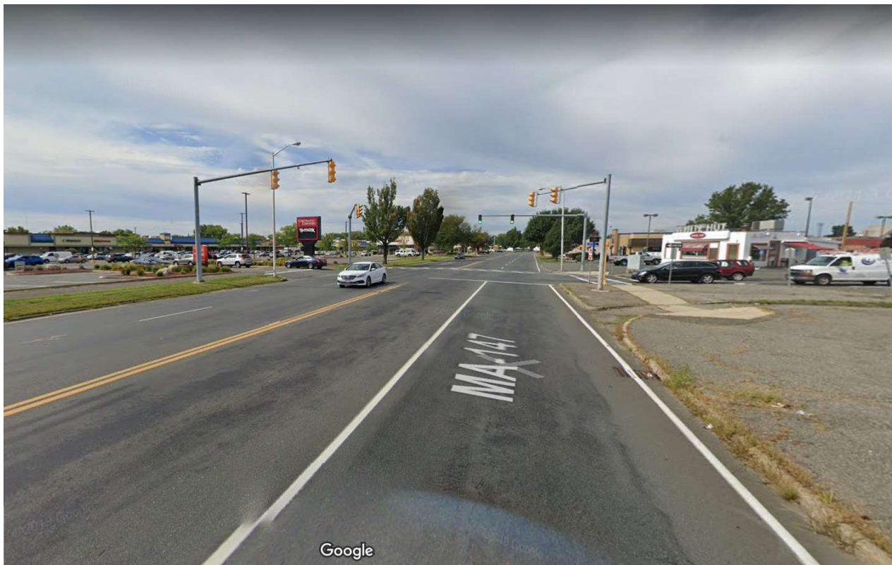
Memorial Avenue (Route 147) approaching Bresnahan Street looking west
